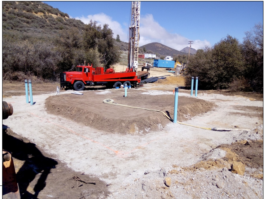
Water Treatment Plant footings and new Montclair well.
