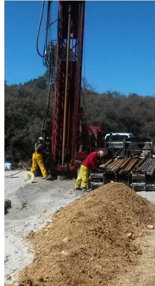
Drilling New Montclair well
